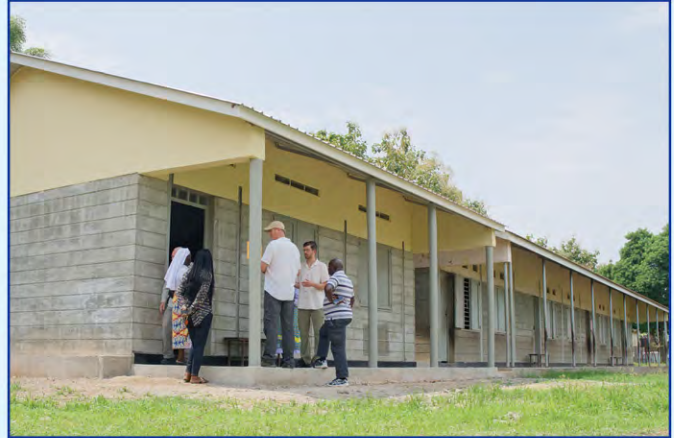
SRF staff inspecting a new school building.
